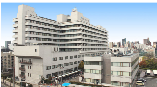
Fig. 1 Exterior of Daini Osaka Police Hospital
